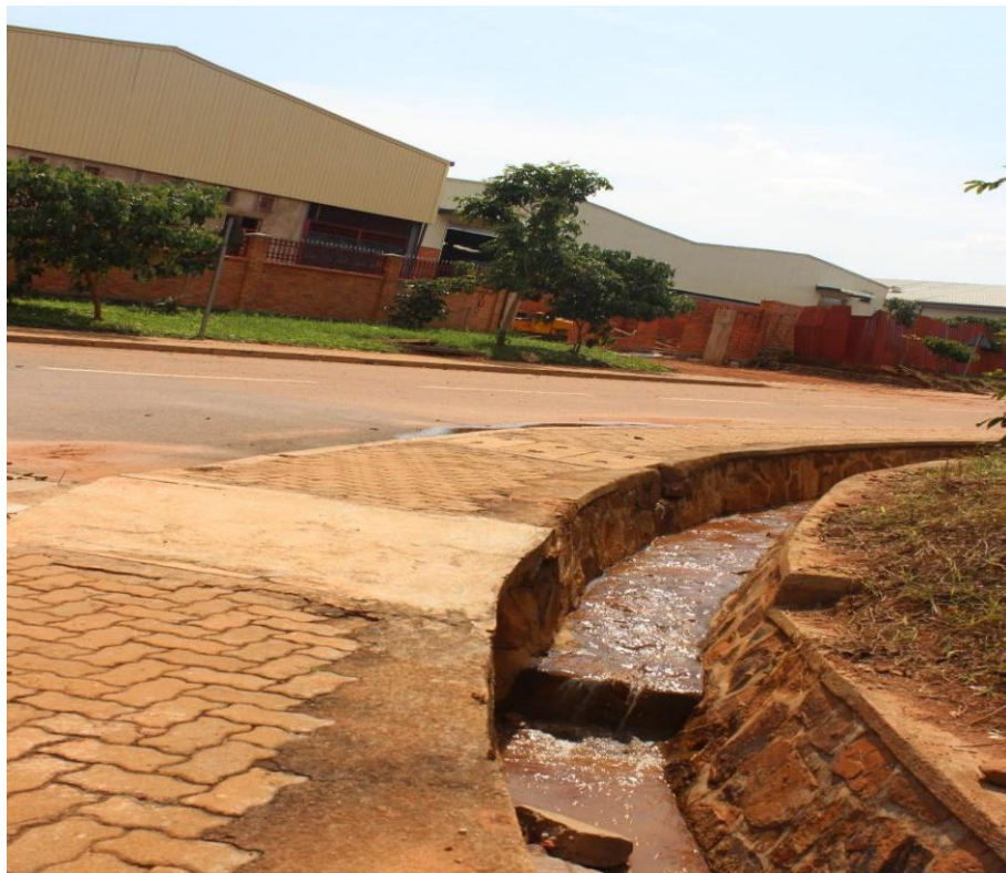
Figure 2:Discharge of wastewater in drainage channel
