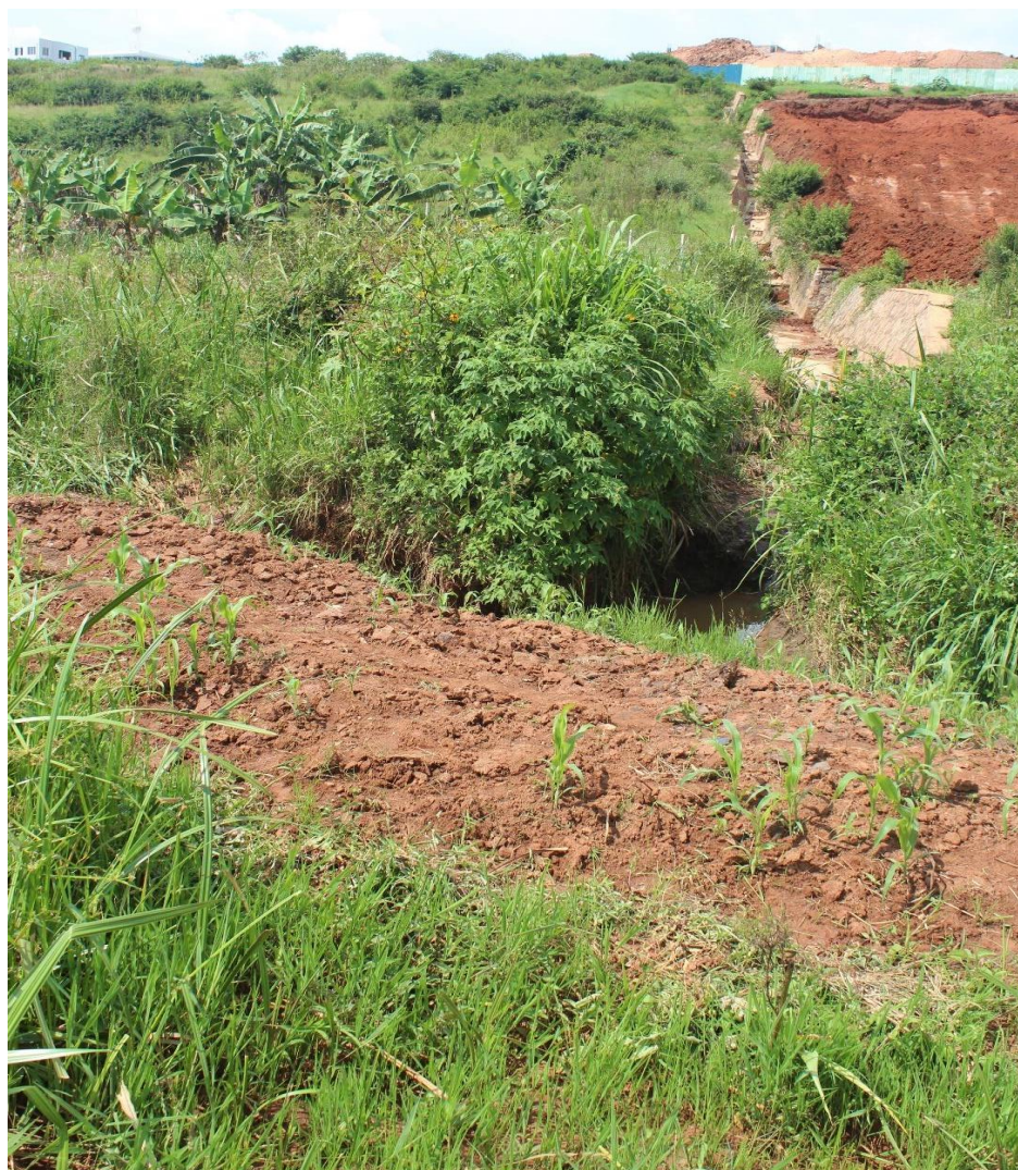
Figure 4: Drainage channel conveying wastewater in the wetland
