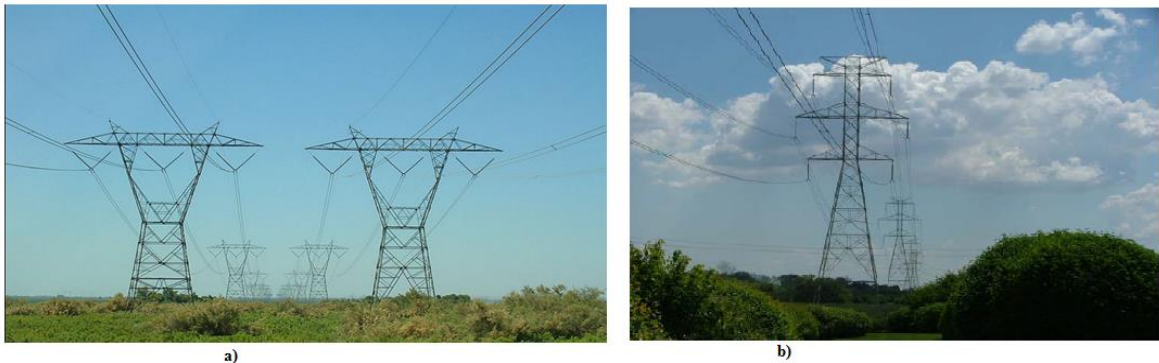
Fig. 3.1 Parallel and double circuit lines
