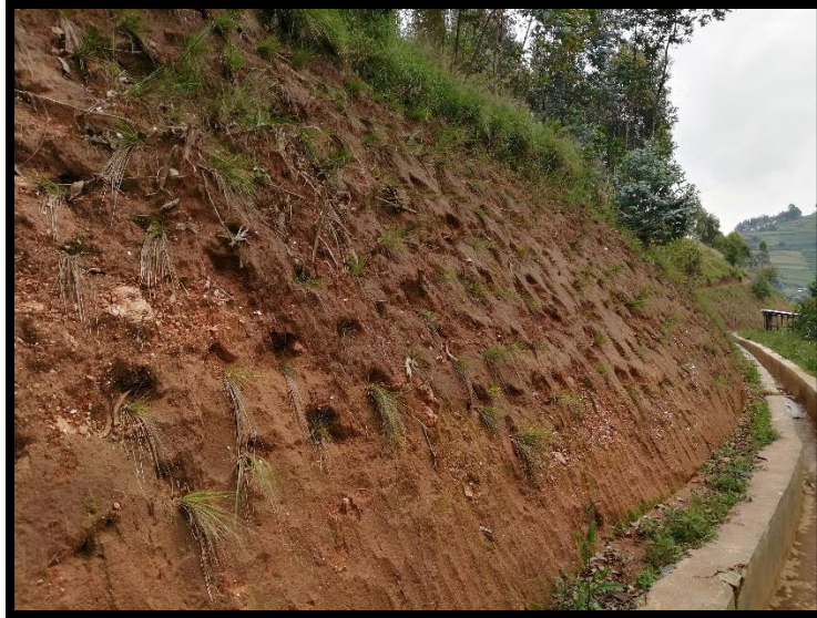
Figure 26: A long canal open channel (Mukwindi,2019)
