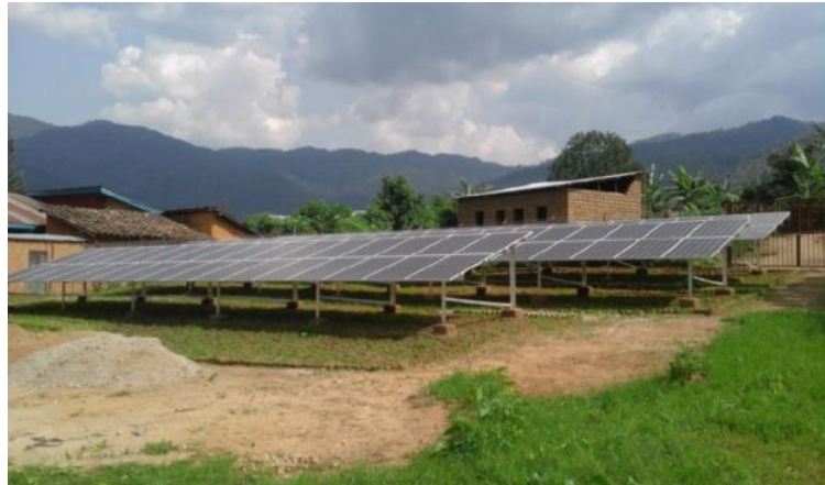
Figure 3: Solar mini-grid for rural village electrification [ Rwanda off-grid status report 2018 ]
