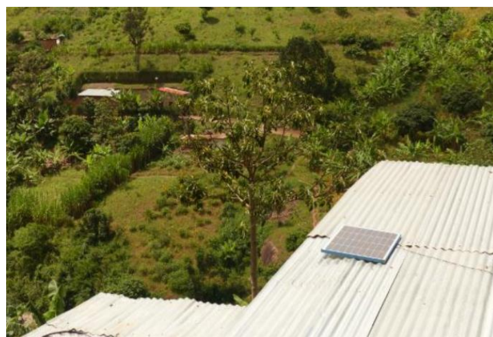
Figure 4:Solar home system [ Rwanda off-grid status report 2018 ]
