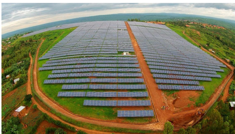
Figure 2: Rwamagana solar power plant [ Rwanda Energy Group ]
