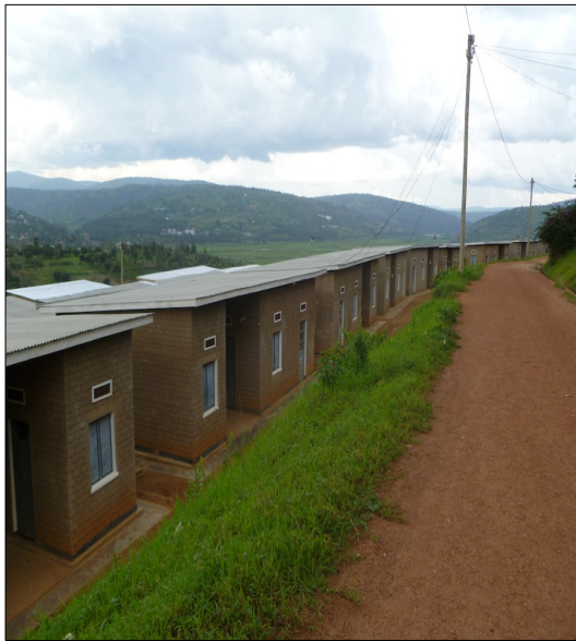
Figure 4.5: Batsinda Estates I. A single affordable housing scheme comprised of 250 units in Kigali. MININFRA (2014).
