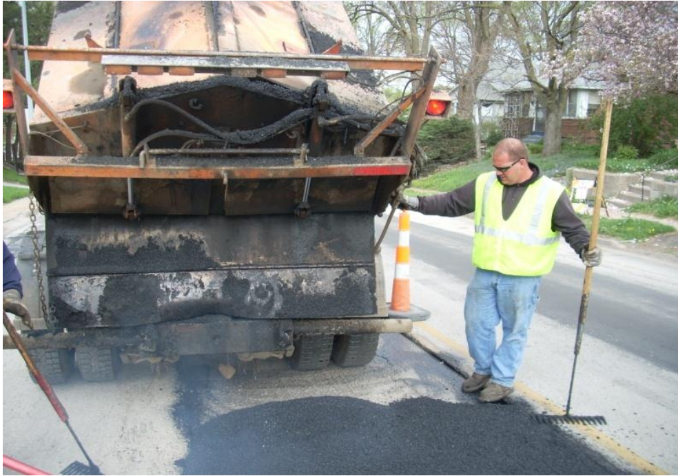
Photo 7: Repair of utility cuts
