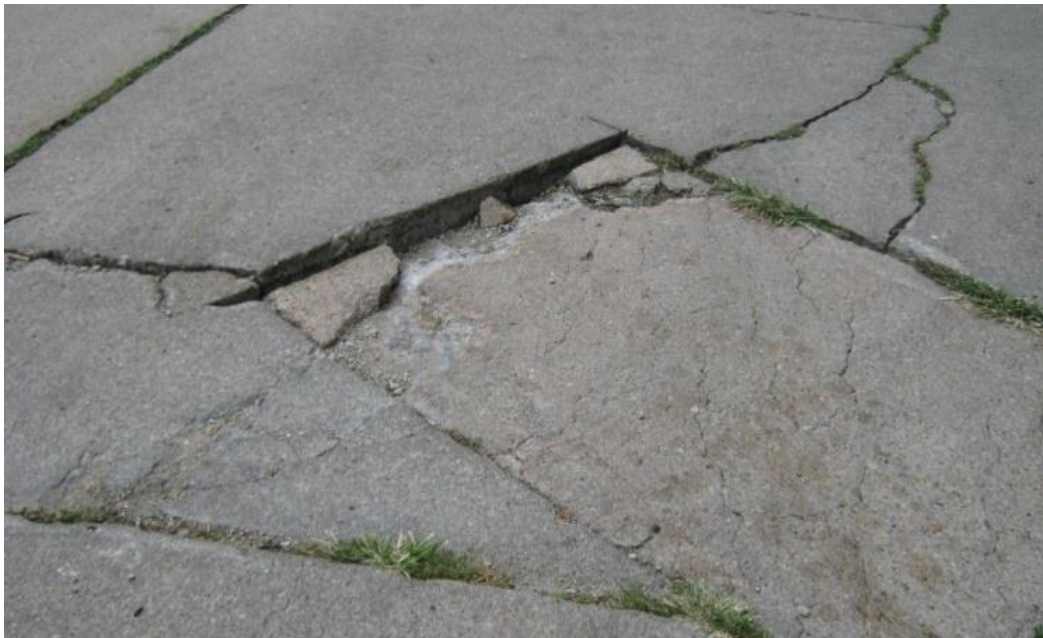
Photo 3: Utility cut, not repaired, with depression
