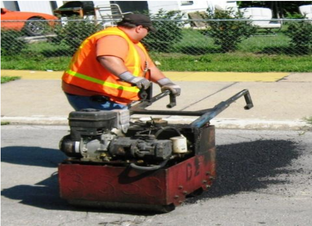
Photo 6: Compaction of asphalt on the utility cuts
