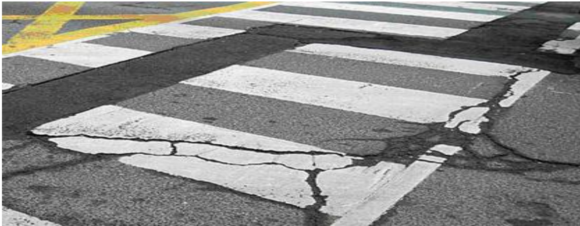
Photo 2: Multiples of repaired utility cuts for different companies bearing pothole, cracks and depressions
