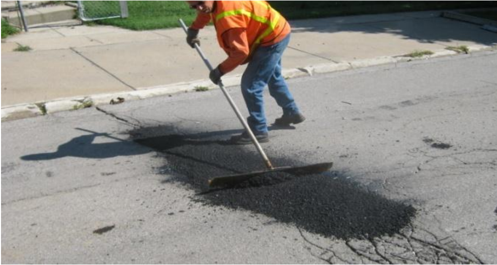
Photo 5: Repairing the utility cuts
