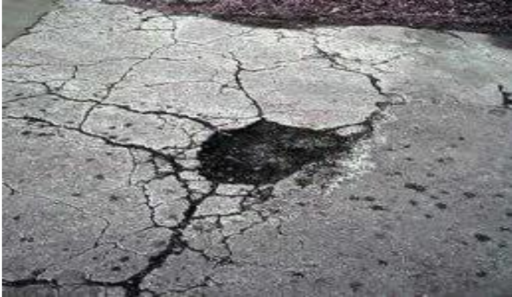
Photo 3: Utility cut, not repaired, with depression
