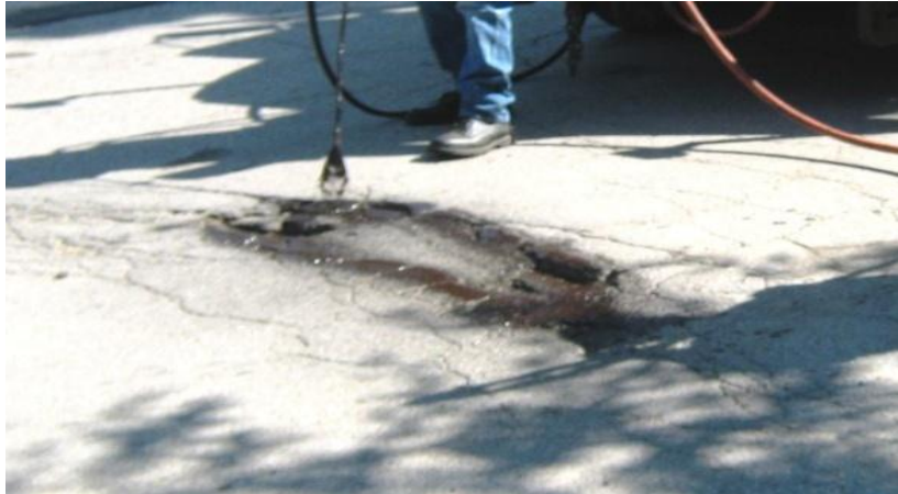
Photo 9: Repaired utility cut with extended pothole and cracks that affect road life and serviceability
