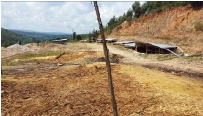
Photo 4-7: General view of one of HABATU active sites
