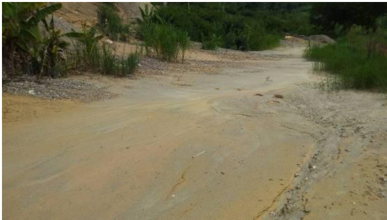
Photo 4-10: Erosion of waste soil at HABATU mine
