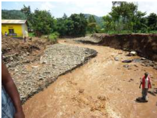
Figure 2 : Katabuvuga river banks destroyed and local people's houses and fields flooded
