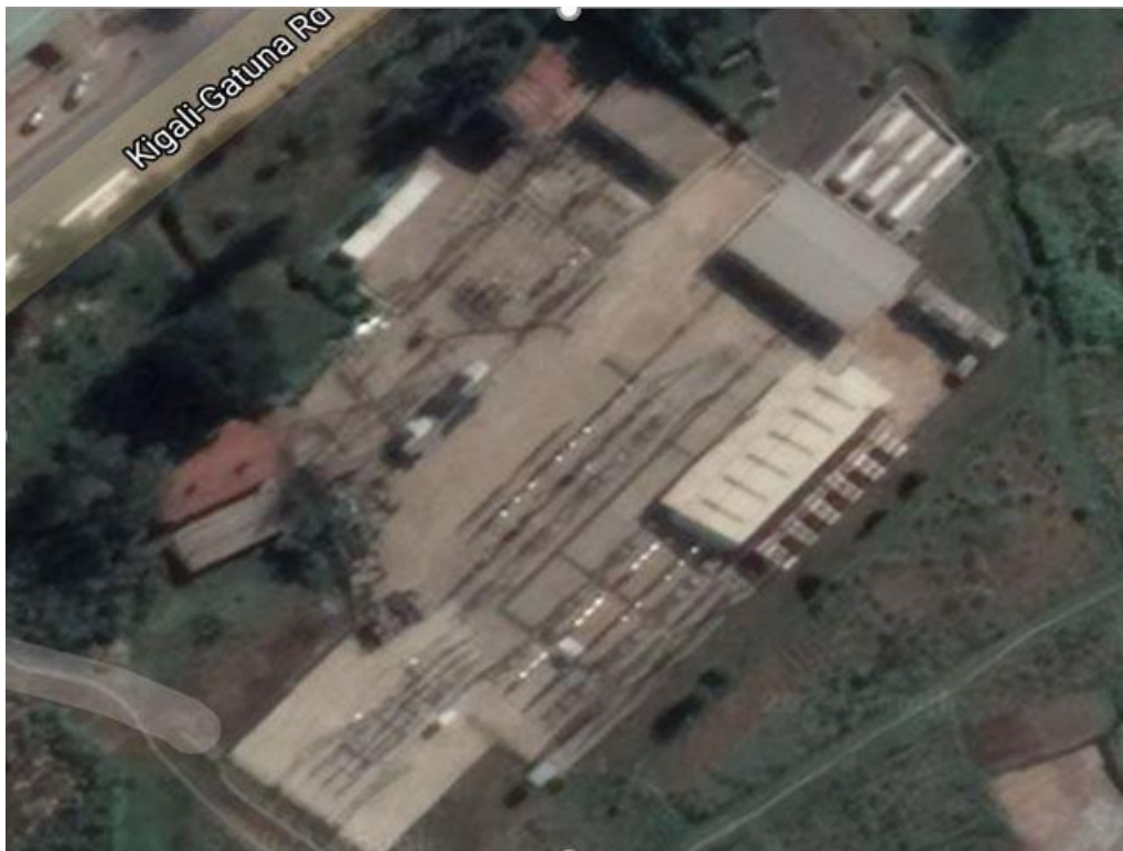
Figure 3. 1: Google map of JABANA Substation
