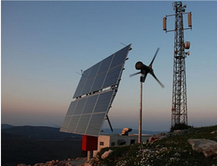
Figure 1. 2 : General PV–wind–diesel powered mobile base station OFF-grid [4].
