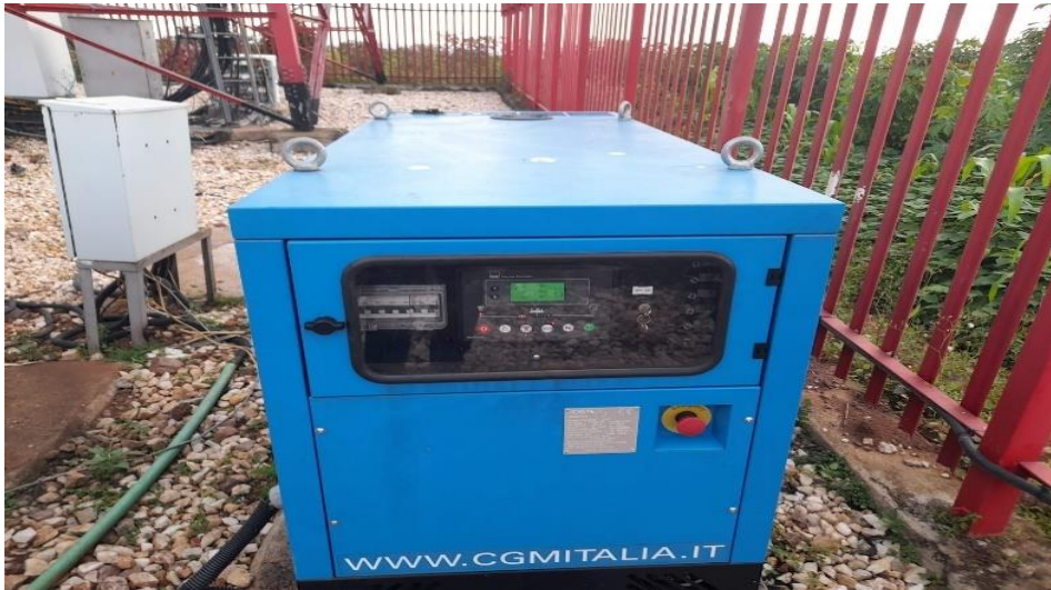
Figure 3. 3: Diesel Generator
