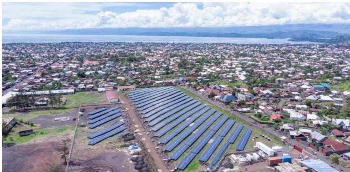
Figure 1.2. NURU solar power plant in Goma city of the DRC.
