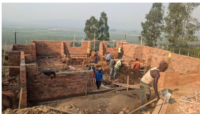
Figure 13: People participating in construction of house earning income
