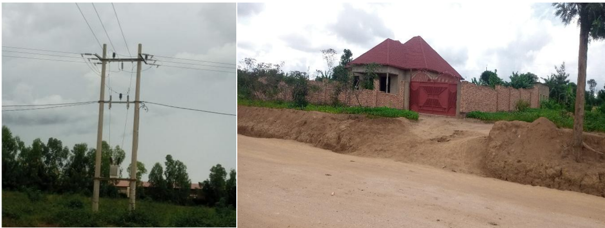
Figure 12: Infrastructure availability in Rilima Sector
