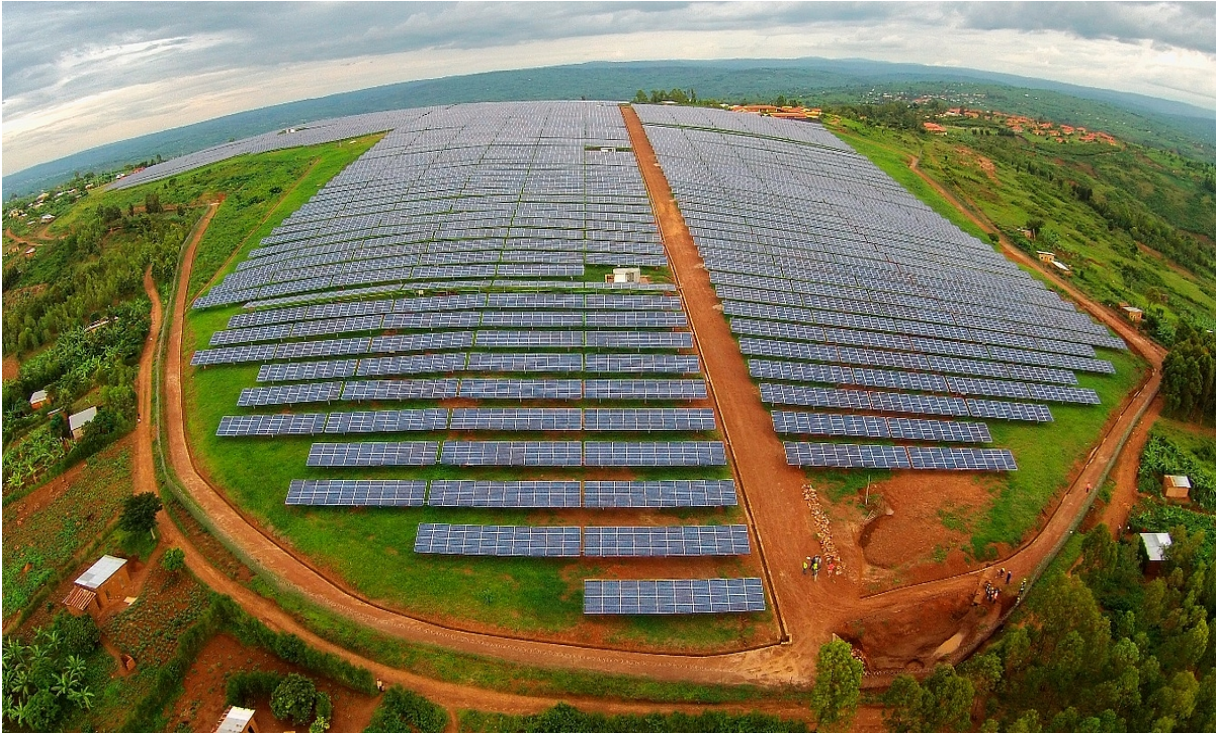
Figure 2-4: Rwamagana Gigawatt generating 8.5 MW
