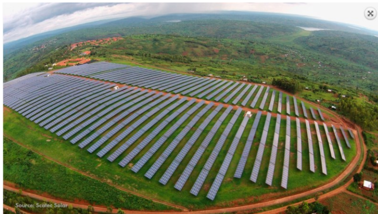
Figure 4. 8:Utility-scale of 8.5MW PV power plant constructed in Agahozo-Shalom Youth Village in Rwanda[57].
