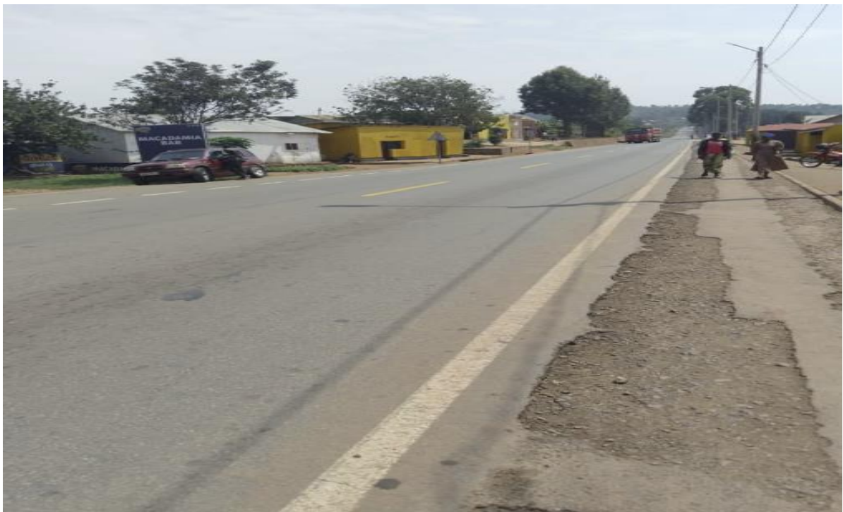
Figure 8: STRAIGHT ROAD SEGMENT AT SHYORONGI WITH GOOD VISIBILITY AND 80KM/H SPEED LIMIT
