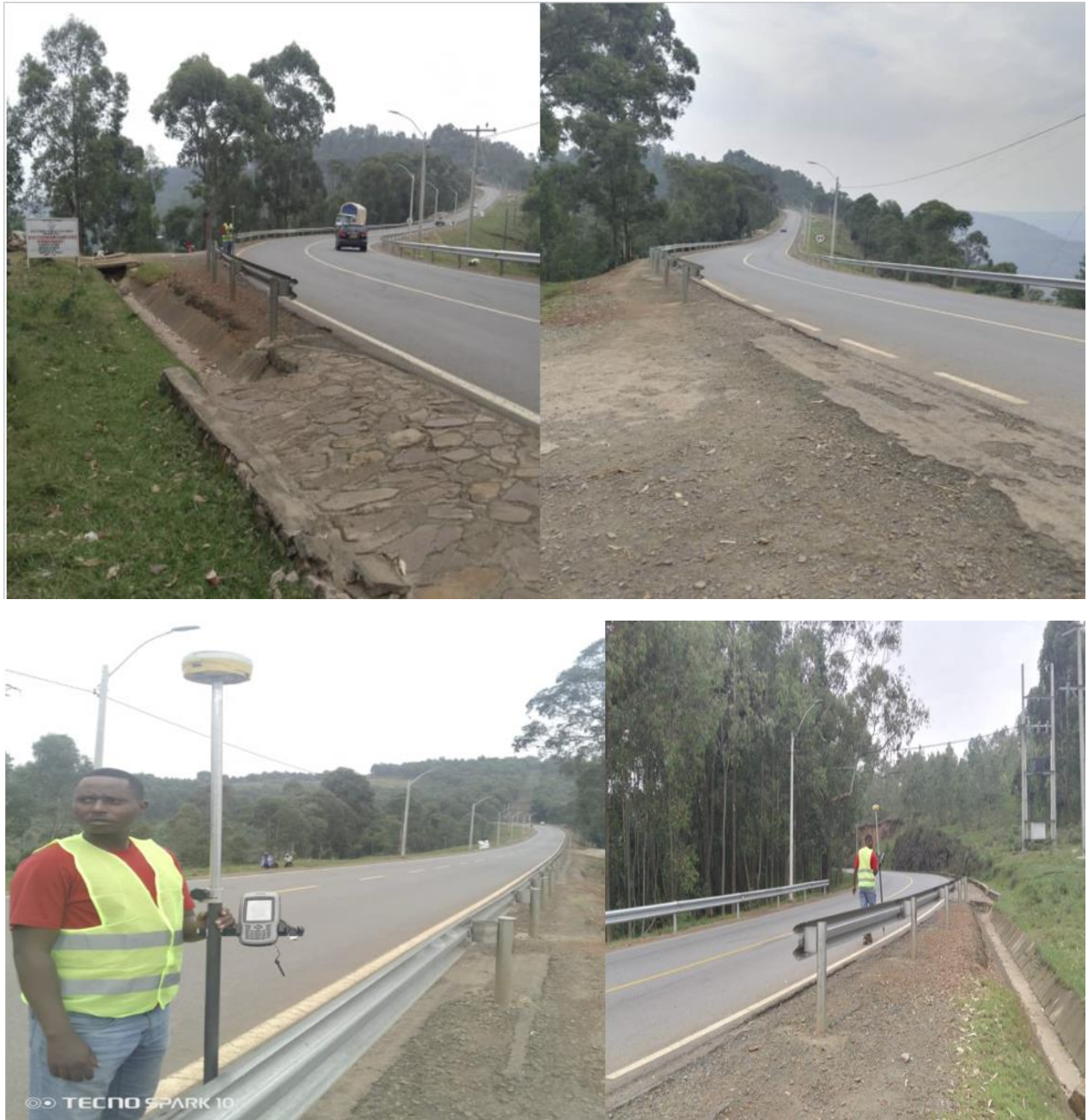
Figure 9: KINGAZI-TABA-RUSIGA SECTOR NEAR KIRENGE CENTER – ACCIDENT-PRONE AREA WITH HIGH FATALITIES IN 2025; SPEED LIMIT IS 80 KM/H. NOTE: BARRIERS WERE RECENTLY INSTALLED FOLLOWING TWO SERIOUS FATAL ACCIDENTS IN 2025.
