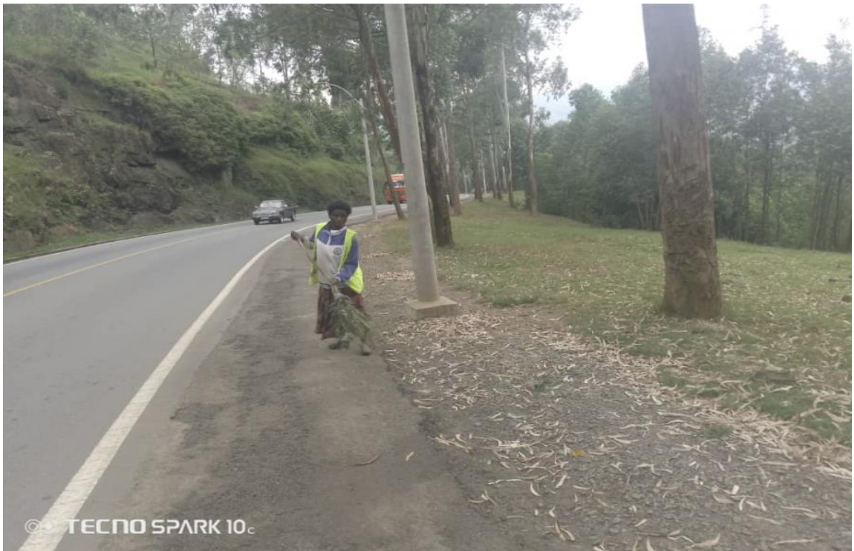
Figure 14: ROUTINE MAINTENANCE ACTIVITY – ROAD CLEANING OPERATIONS
