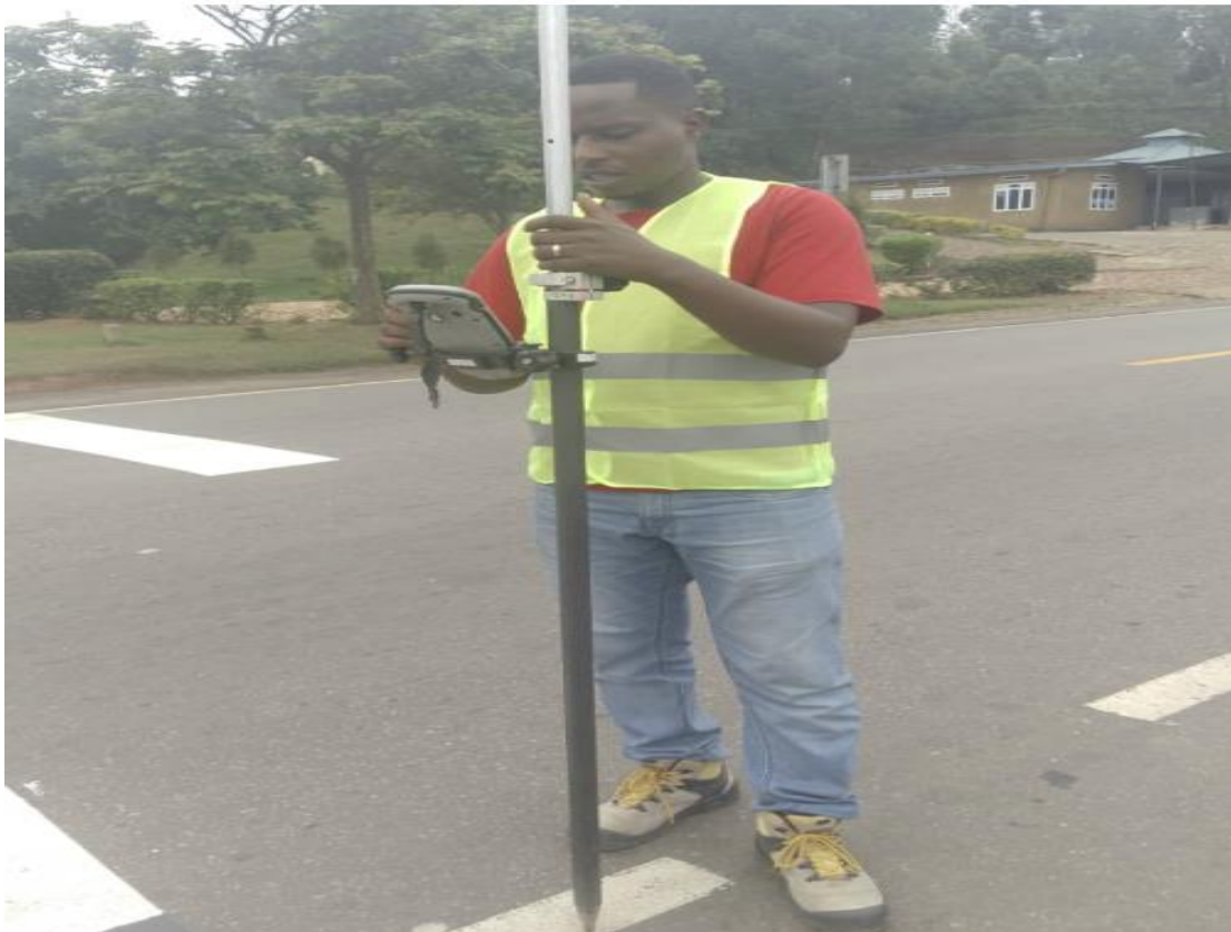
Figure 5: SETTING UP DI-GPS INSTRUMENT FOR DATA COLLECTION ALONG THE ROAD CORRIDOR
