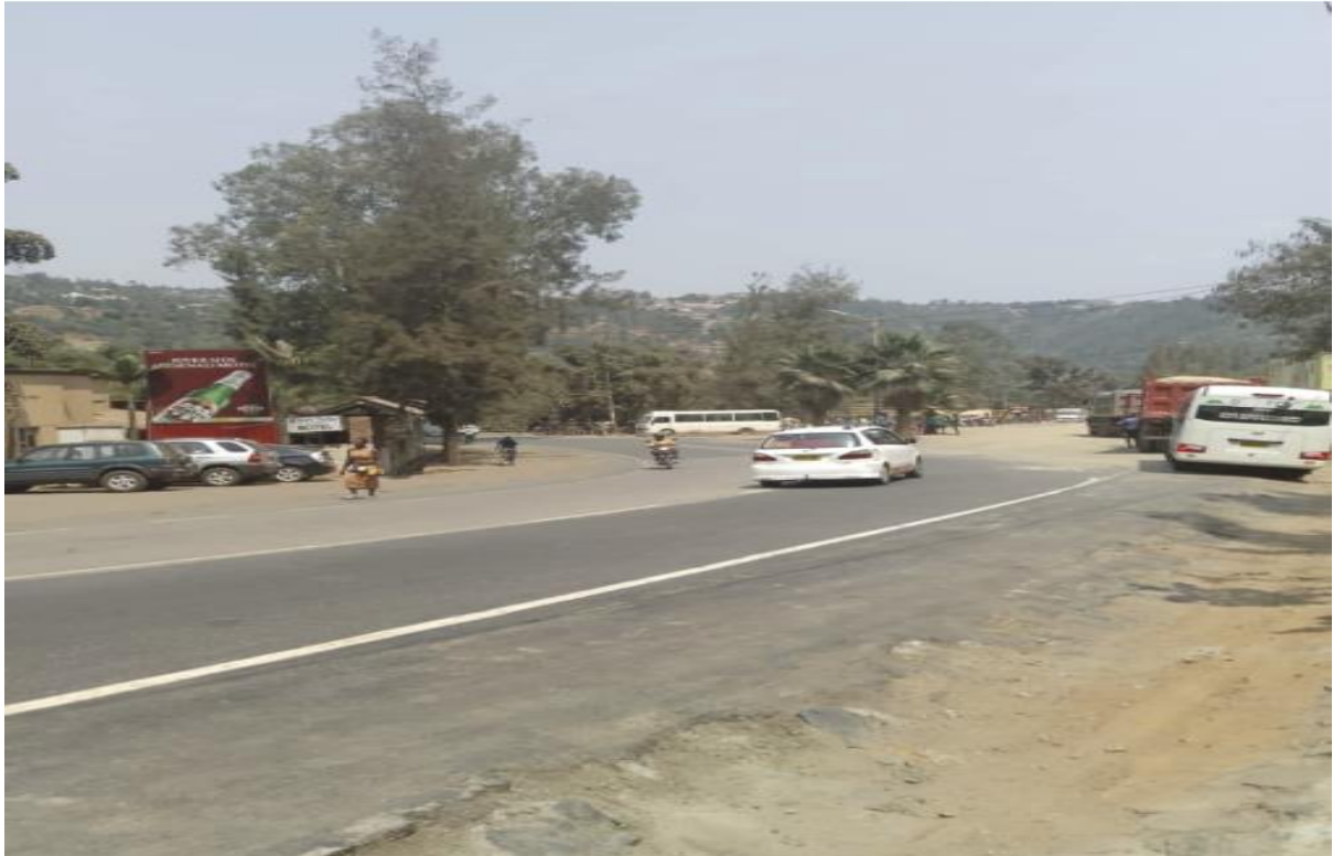
Figure 3: ROAD SEGMENT 2 IMMEDIATELY AFTER GITIKINYONI BRIDGE
