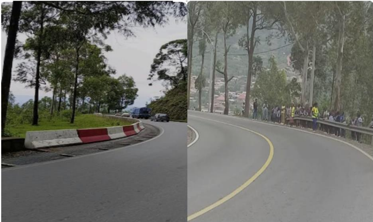
Figure 18: ROAD SAFETY BARRIERS INSTALLED AT HIGH-RISK SECTIONS
