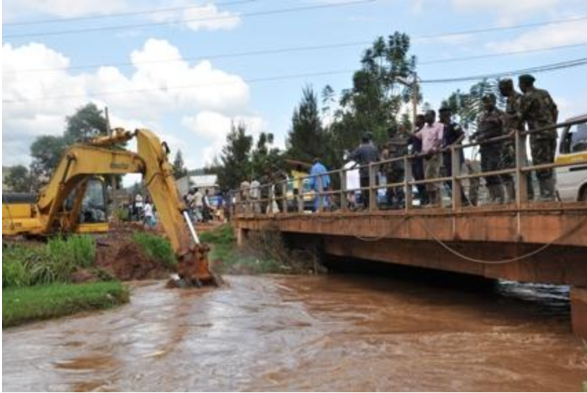
Photo 6: Dredging of the Nyabugogo River
