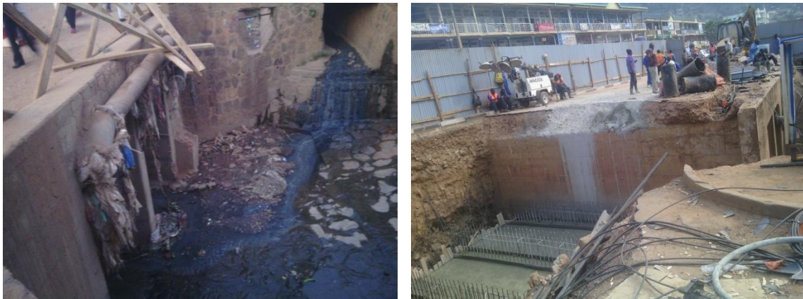
Photo 8: Existing culverts under the bridge on the Road Nyabugogo-Muhima-Town Center
