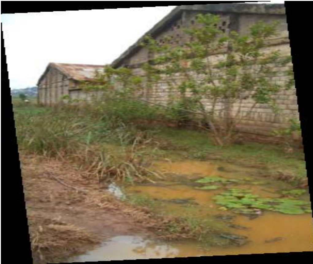
Figure 2.2 : Abandoned warehouse in the Nyabugogo wetland(REMA,2006)
