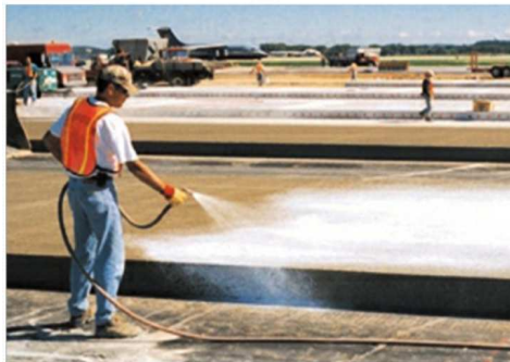
Figure 2.10 Application of concrete curing compound
