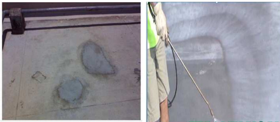
Figure 2.8 Application of external self-curing concrete
