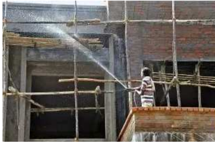
Figure 2.3 Spraying water curing
