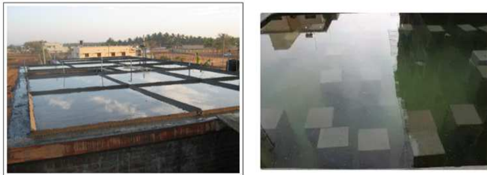
Figure 2.2 Ponding and immersion water curing
