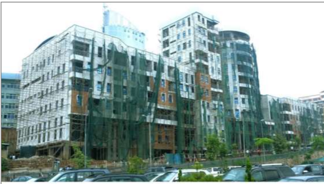
Photo 2: Modern building under construction Source: Field survey
