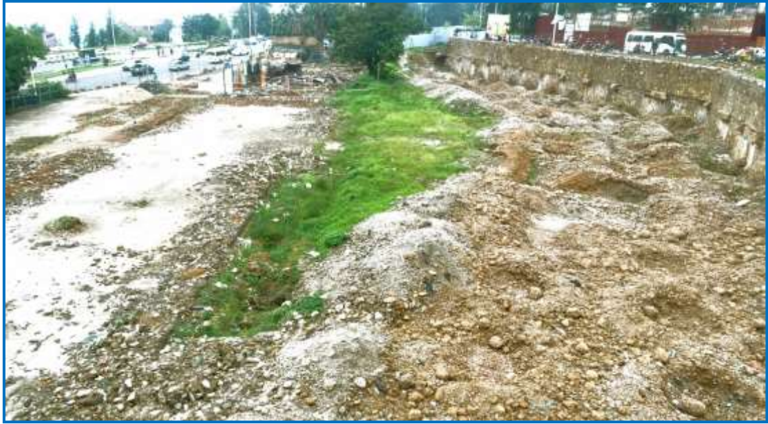
Photo 1: Area of land where houses were demolished Source: Field survey
