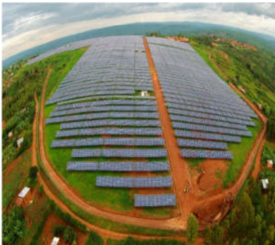
a) The 8.5 Megawatt (MW) power plant in Rwanda located in Rwamagana [14]
