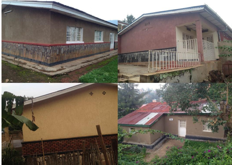
Figure 25. Site photo 6 showing different materials for the facades
