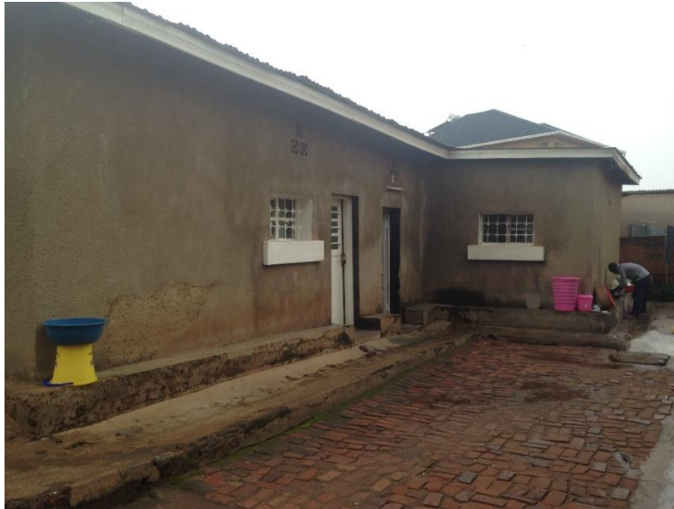
Figure 24. Site photo 5 showing the outdoor area
