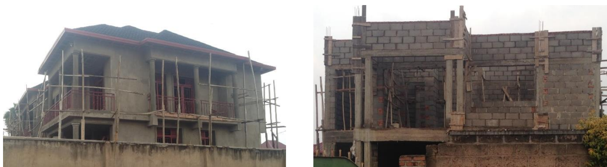
Figure 18. Site photo 5&6 showing renovations
