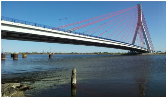
Inverted Y-Type, Third Millennium John Paul II Bridge, Poland ( source: https://en.wikipedia.org )
