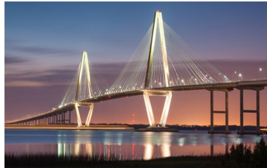
Diamond-Type, Arthur Ravenel Bridge, South Carolina ( source: https://en.wikipedia.org )
