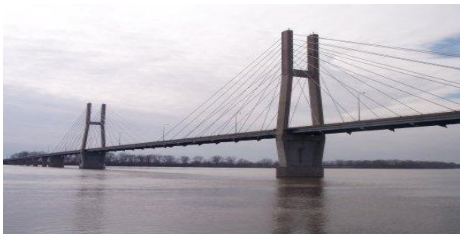
Figure 3.3. Quincy Bayview Bridge 8
