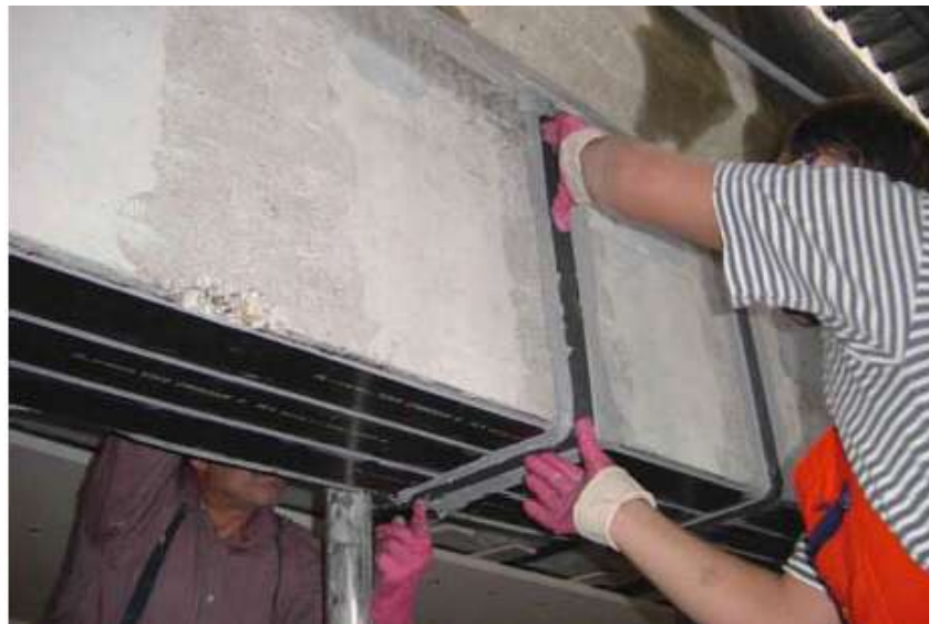
Figure 1.1: Typical application of FRP plates on RC beam (Motavalli & Czaderski, 2007)
