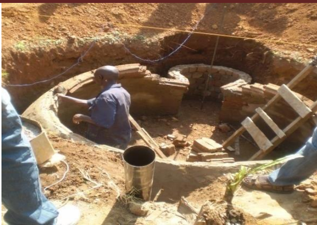
Figure 18: Construction of biogas plant (CAMARTEC model)
