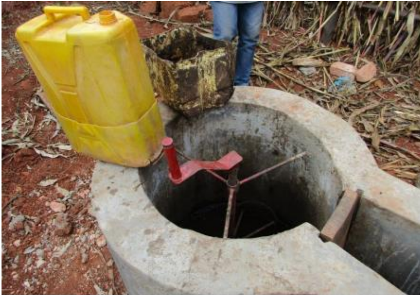
Figure 17: Biodigester inlet
