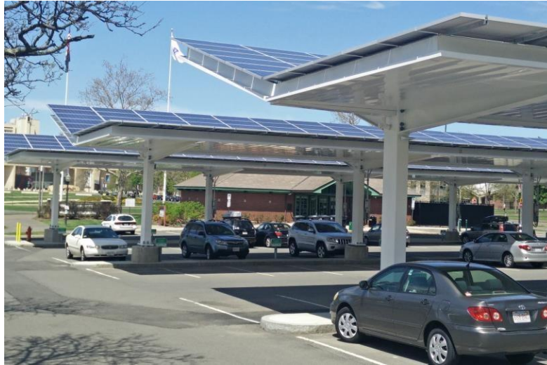
Figure 14: solar parking lots chargers
