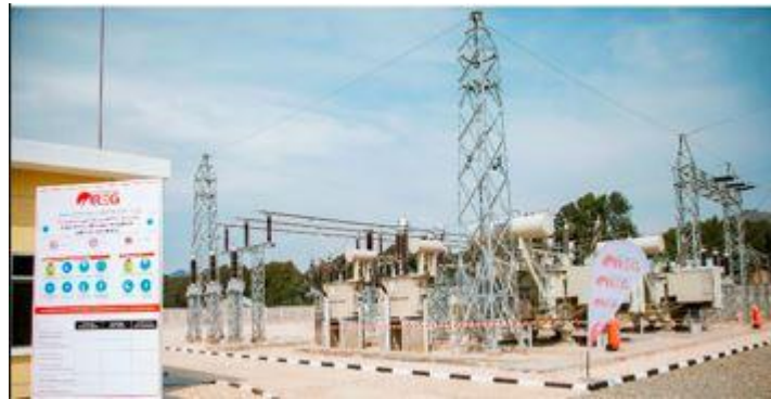
Figure 25: distribution substation
