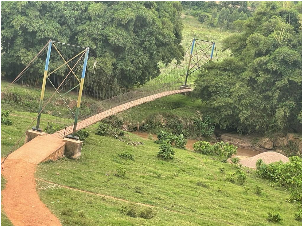
Figure 2:Nyirakibehe suspension bridge (Source: Taken by myself).
