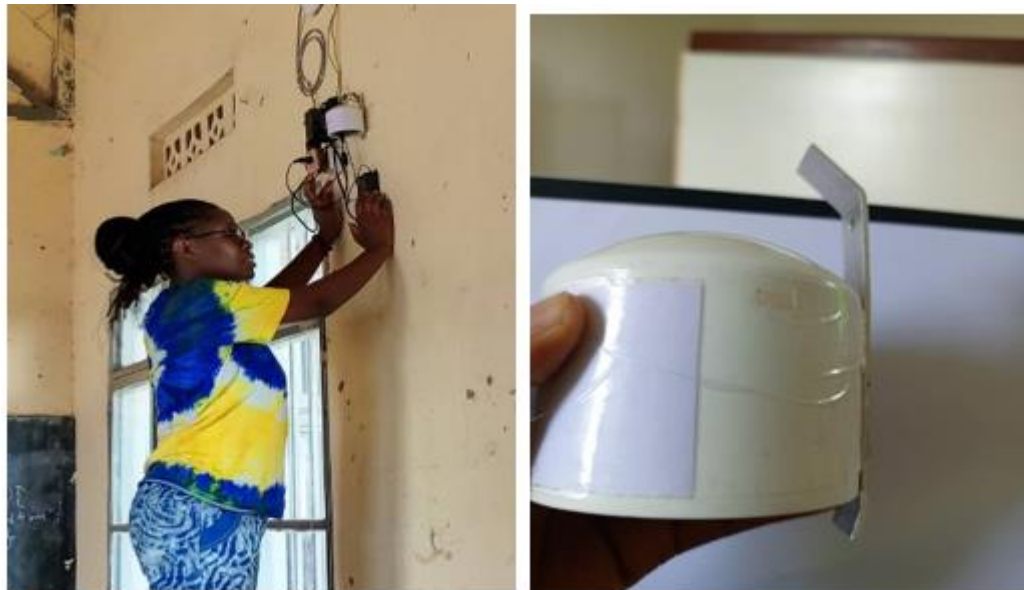
Figure 5: Photo showing the installation of the Purple Air Sensor. (Source: Photograph, 2023)
