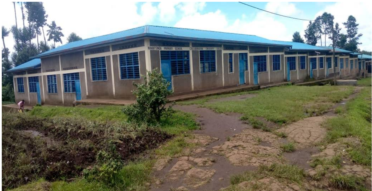
Figure 3: Nyabitsinde Primary school in Kinigi Sector
