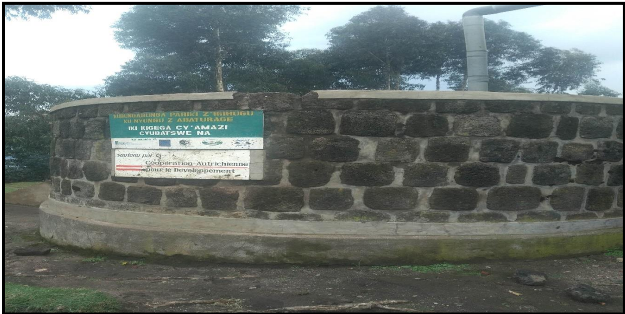
Figure 6: Water tank constructed by TRS funds in Gataraga Sector
