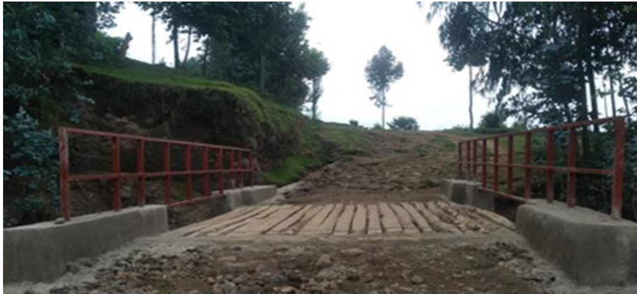
Figure 10: Bridge infrastructure constructed by TRS funds in Gataraga Sector
