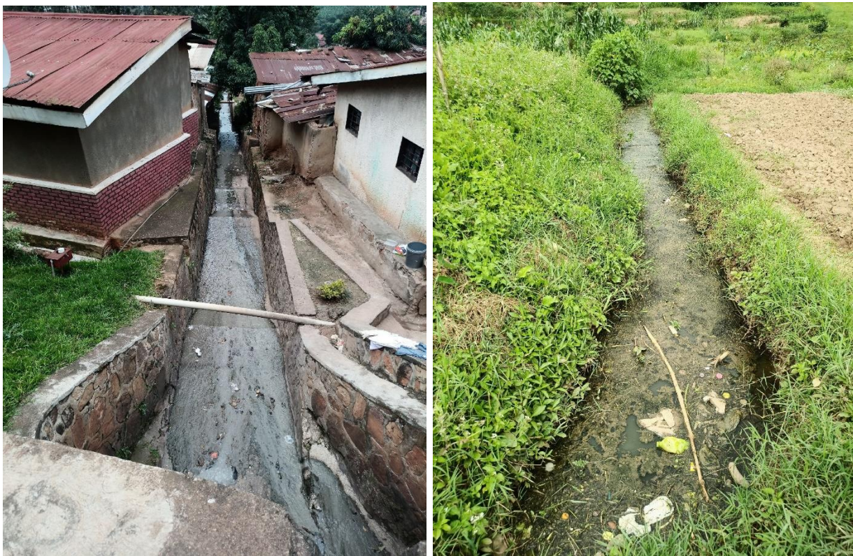
Figure 11. Open drainage & Drainage that flows toward wetland (Source: Field survey)
