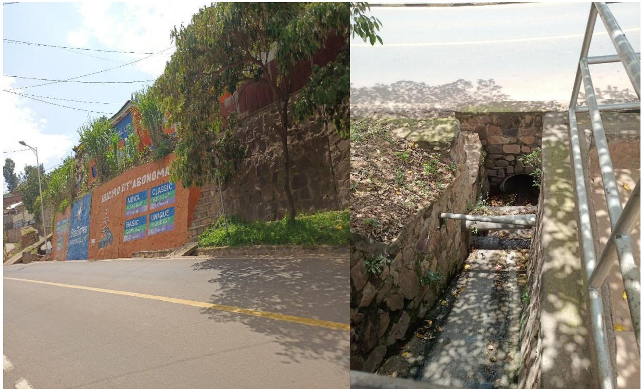
Figure 15. Retaining wall and guardrails for protection (Source: Field survey)
