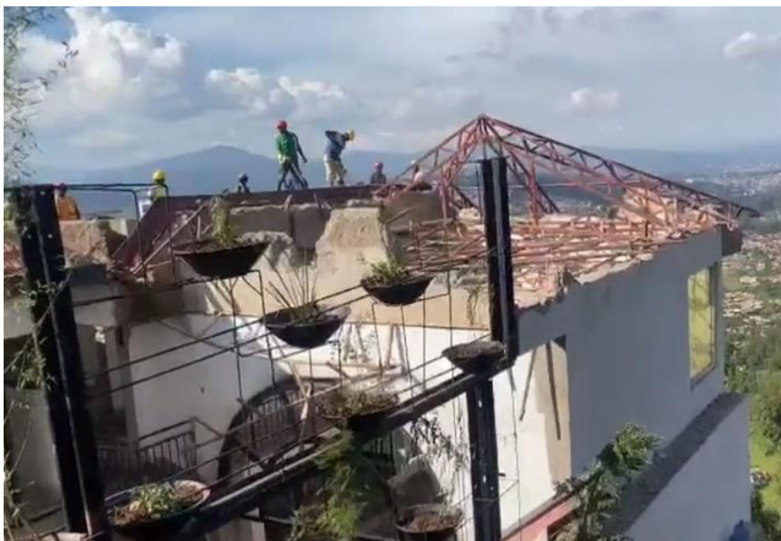
Figure 2-1: A hotel top floor being demolished Source: Kagire (2023)
