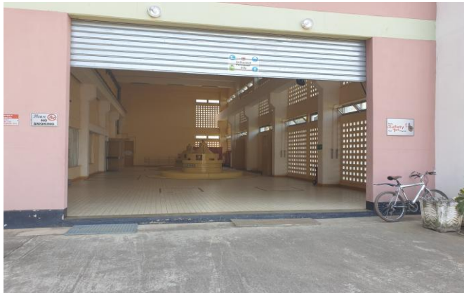
Figure 2: Mukungwa 1 HPP power house
