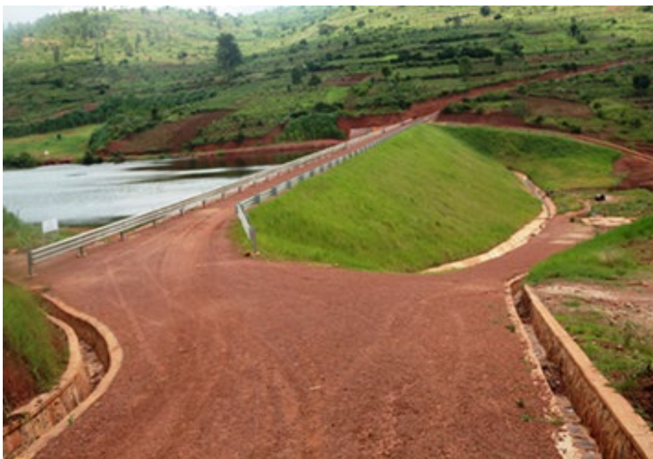
Figure 4.6: dam with water canals for dam protection
