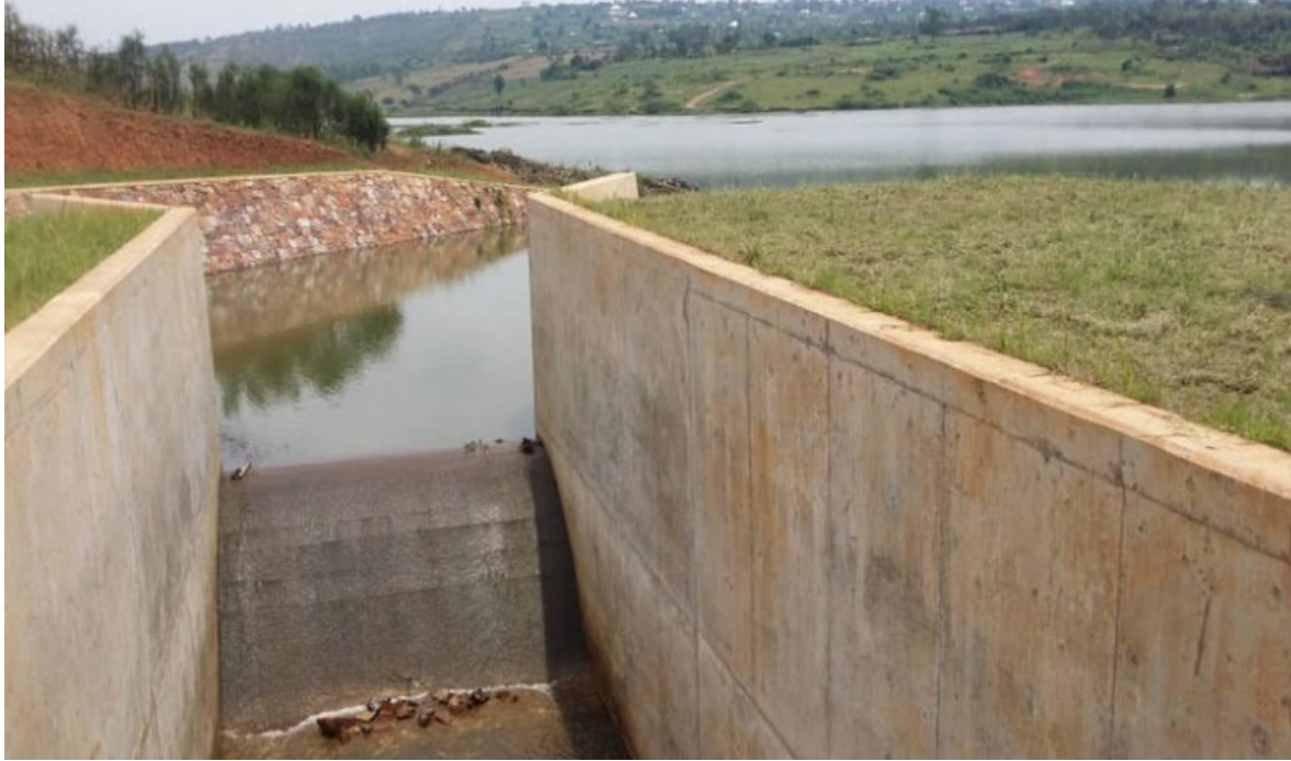
Figure 3.4: the new dam for irrigating crops at Cyaruhogo wetland (Bugugu dam)
