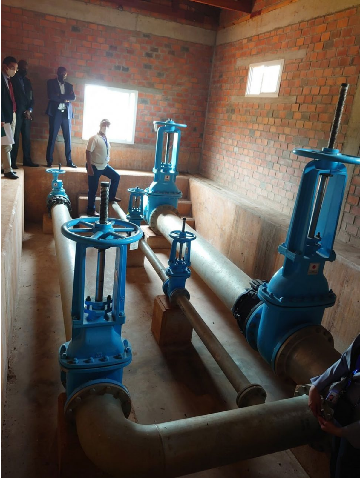
Figure 3.5: modern in the irrigation infrastructure of Cyaruhogo wetland
