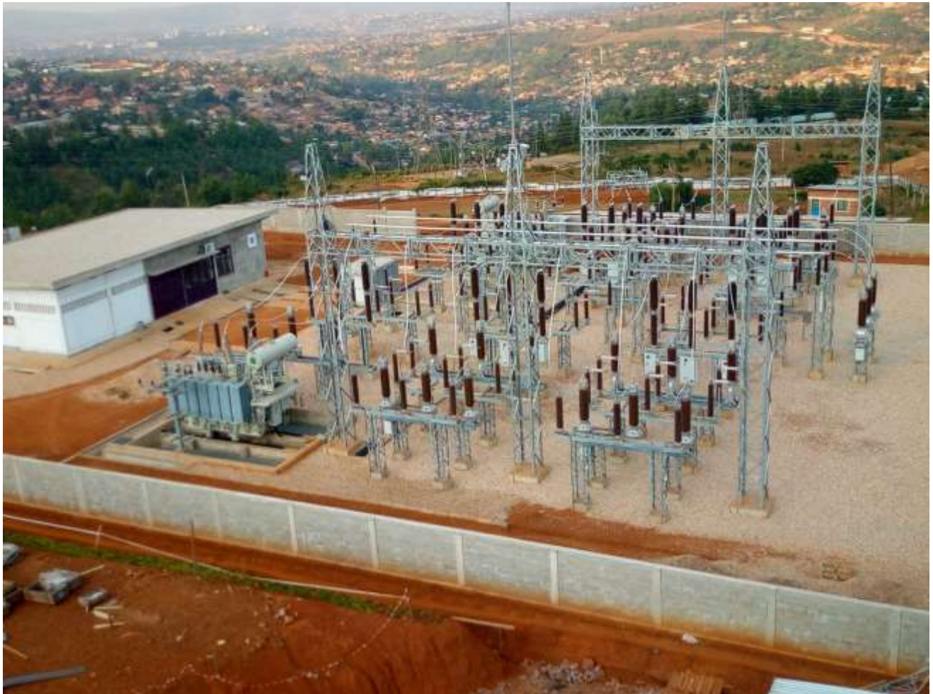
Figure 8 Photo Image for Mont Kigali Substation
