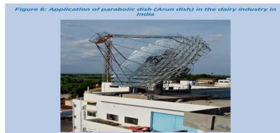
Figure 2-10: Application of parabolic dish in a dairy industry in India [18]
