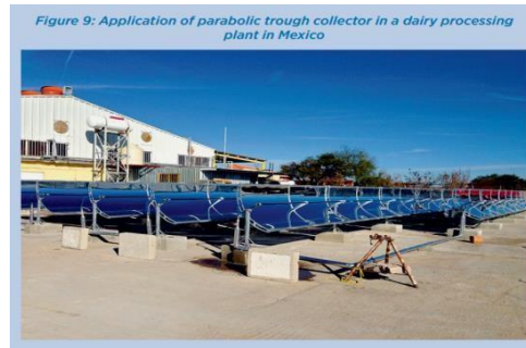
Figure 2-8: Application of PTC in a dairy processing plant in Mexico [18]
