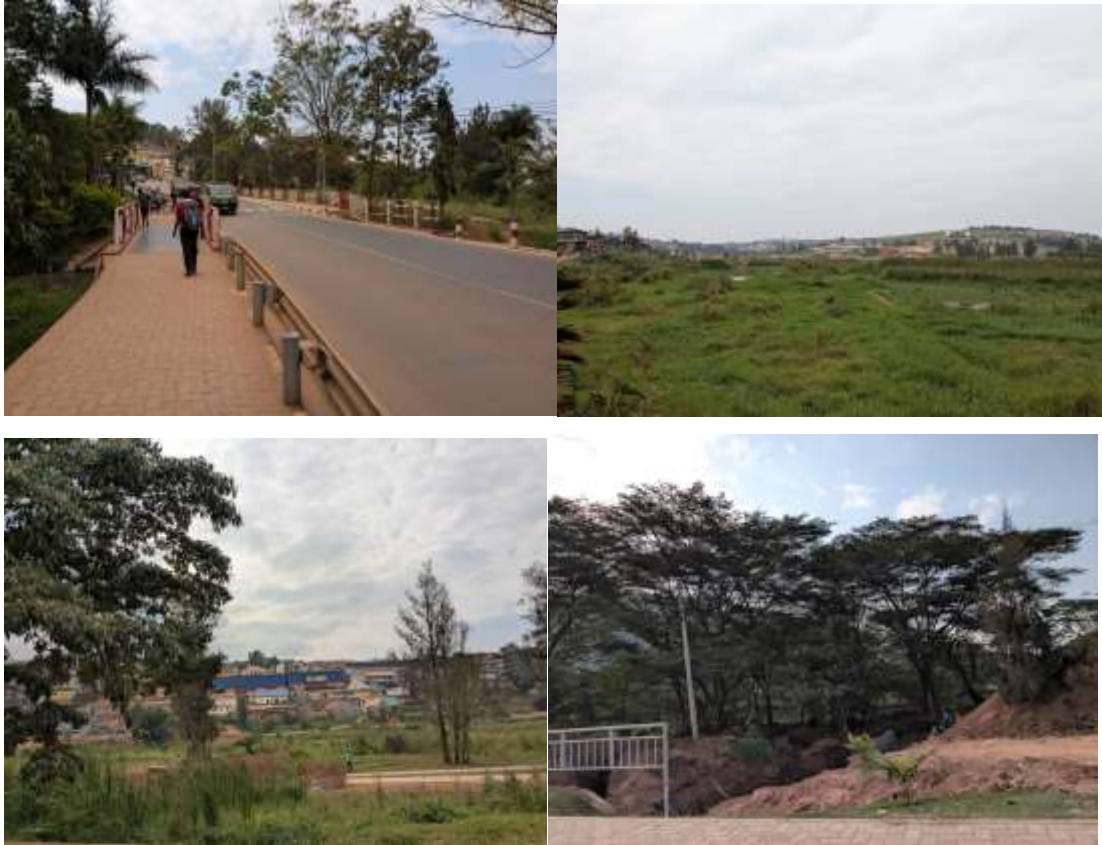
Figure 10: Right up Kinamba bridge. Left up view of Kibumba wetland from Gakinjiro. Right down Kibumba wetland rehabilitation. Left down Nyabugogo wetland rehabilitation
