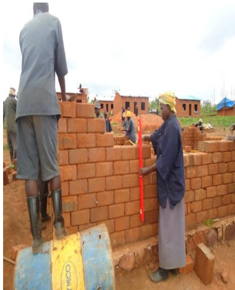
Picture no3: Masonry
