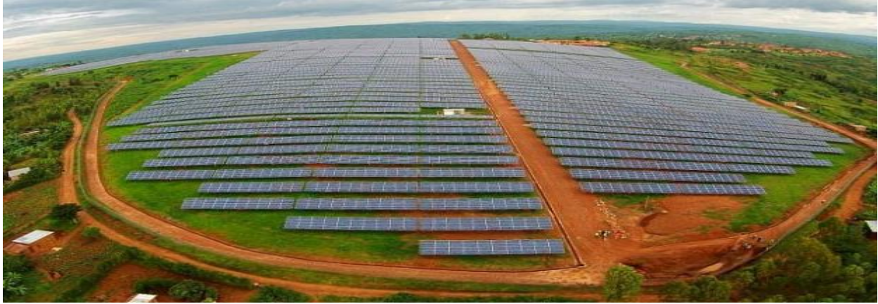
Figure 2.1: Utility scale of 8.5MW PV power plant constructed in Agahozo Shalom Youth Village in Rwanda
