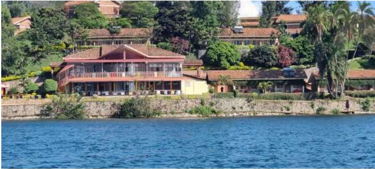
Figure 16: Built up area in the buffer zone of Lake Kivu (Source: Author, 2023).
