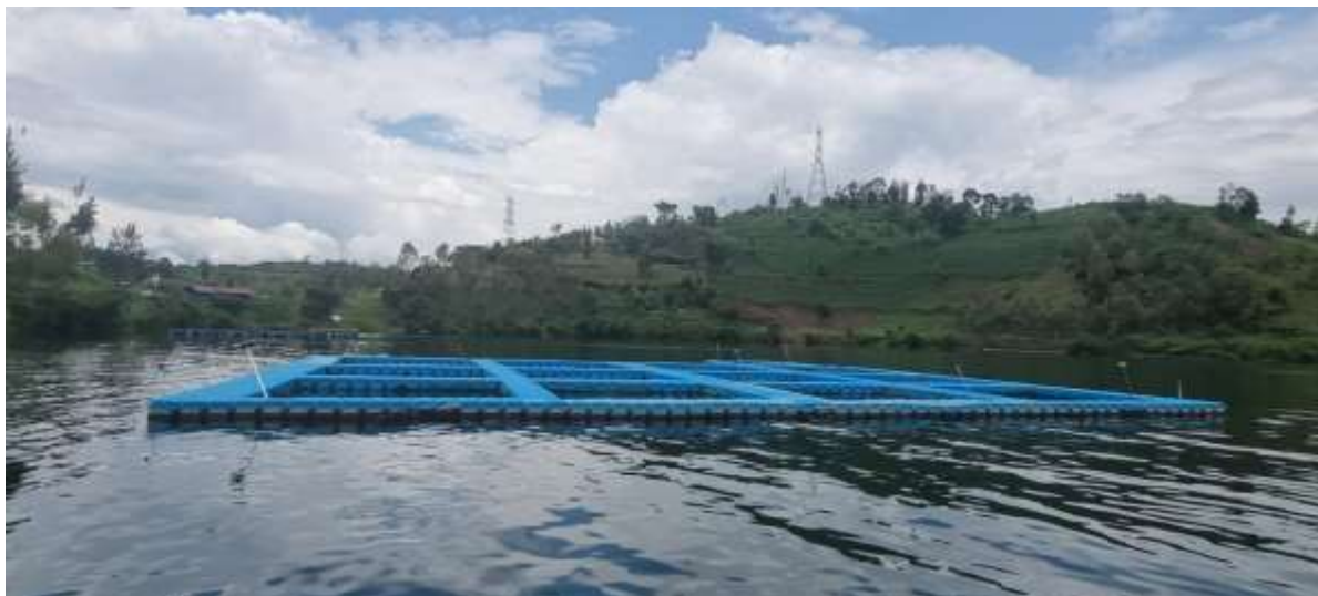
Figure 4: Floating system made of plastic pontoon cubes (Source: Author, 2022).
