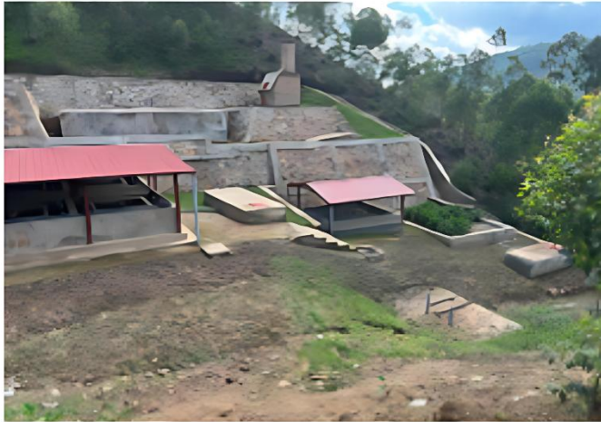
(A) General overview of the plant
