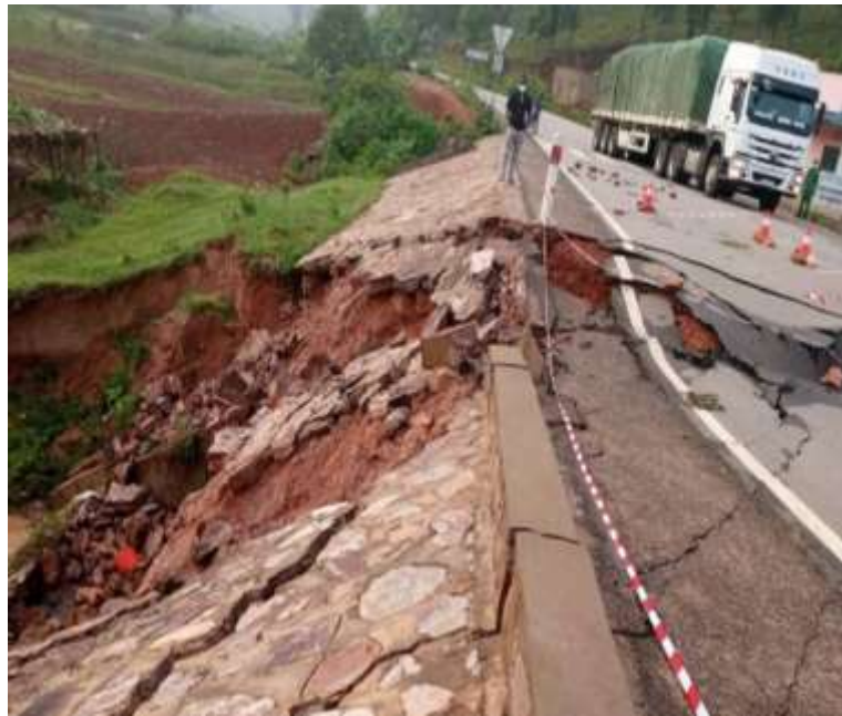
Figure 1- 1 The Failure of Road Huye-Nyamagabe at Nkungu near Nyamagabe Town
