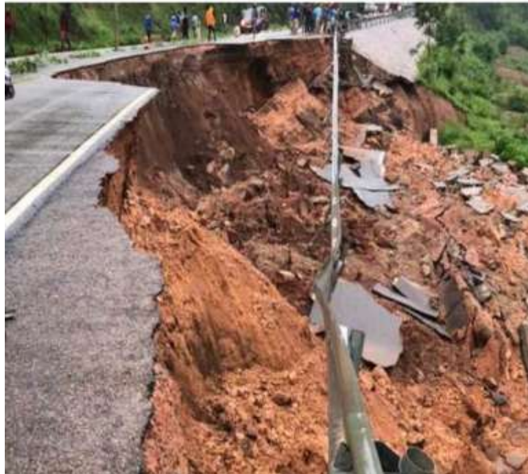
Figure 1- 2 The failure of road Huy heavy rains in Karambi cell, Kigoma sector in Huye district(NKURUNZIZA, 2024).
