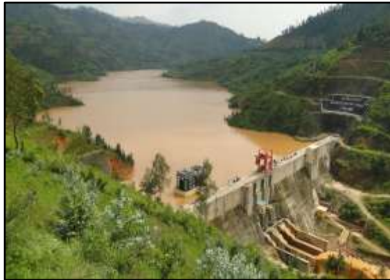
(c) Nyabarongo HPP dam view
