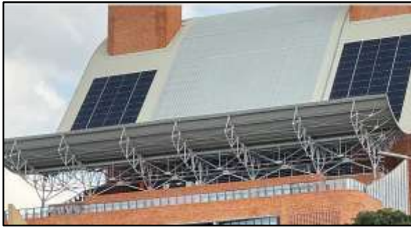
(a) Roof mounted SPV at I & M Bank/Rwanda
