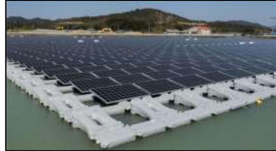
(f) Floating solar PV
