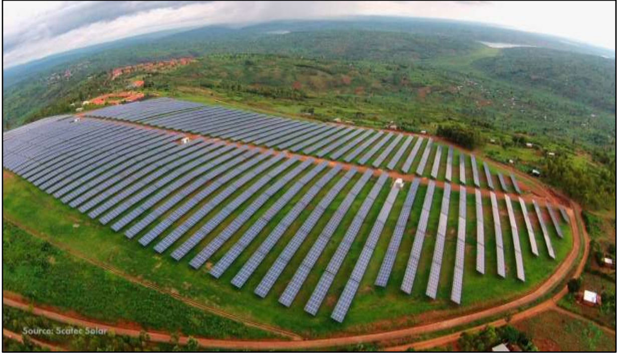
Figure 1. 2: Utility-scale of 8.5 MW PV power plant constructed in Agahozo-Shalom Youth Village [4]
