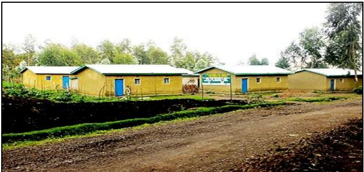
Figure 7: Part of the Kinigi Village built by SACOLA (Photo R. Kabanda, 2013).
