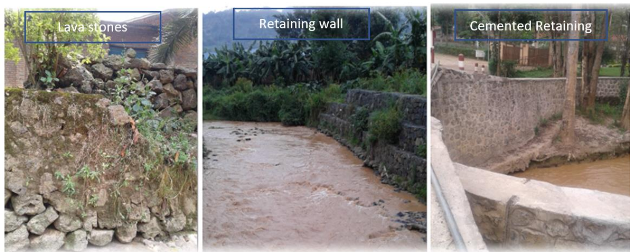
Figure 15: Structural techniques for flood resilience
