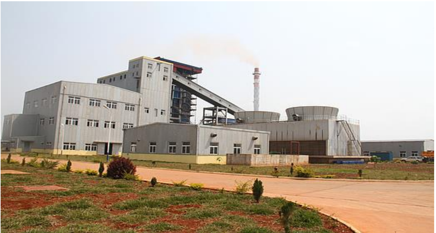
Photo 1:Gishoma Peat Power Plant (REG web site on 31 May 2017
